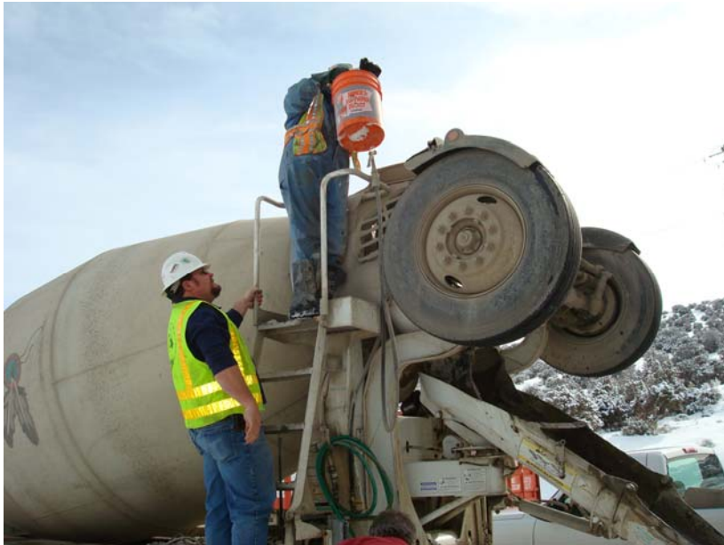
Fig. 4. TOXECON™ ash added during concrete mixing.
