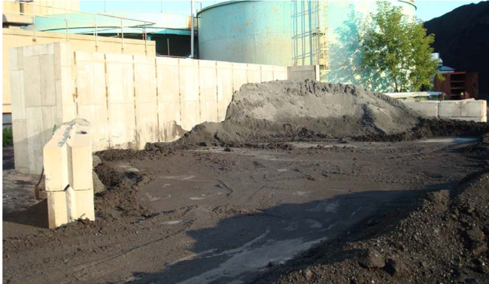
Fig. 12. High-carbon concrete pad used for bottom ash dewatering.
