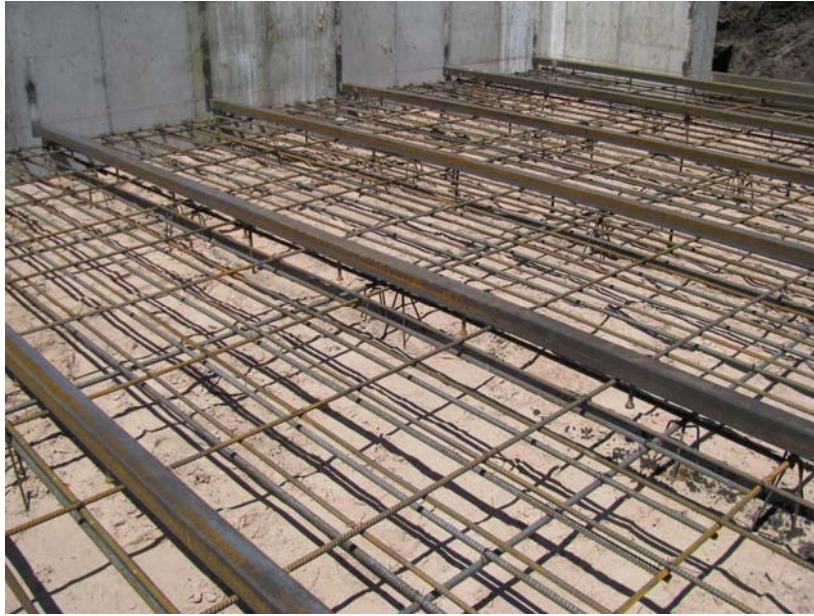
Fig. 6. Completed push wall and support steel for high-carbon concrete pad.
