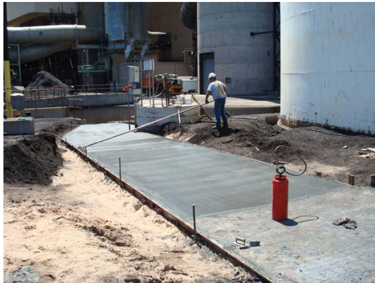
Fig. 9. Completion of the drainage area with high-carbon concrete.
