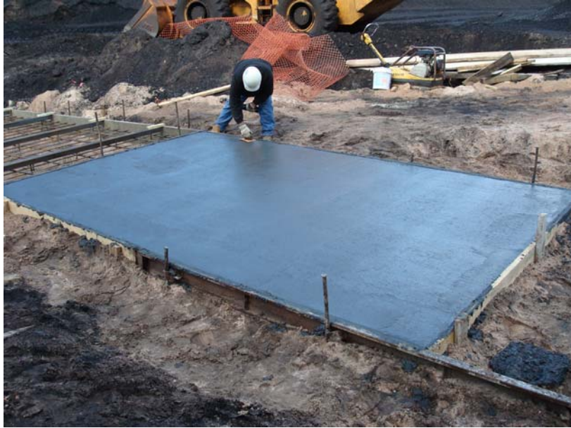
Fig. 8. First successful high-carbon concrete placement.
