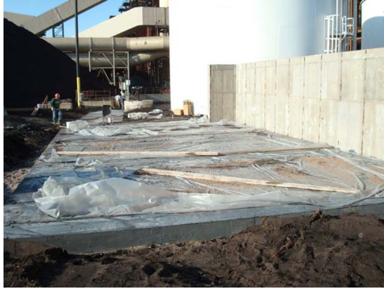
Fig. 10. Completed high-carbon concrete pad after the forms were removed.
