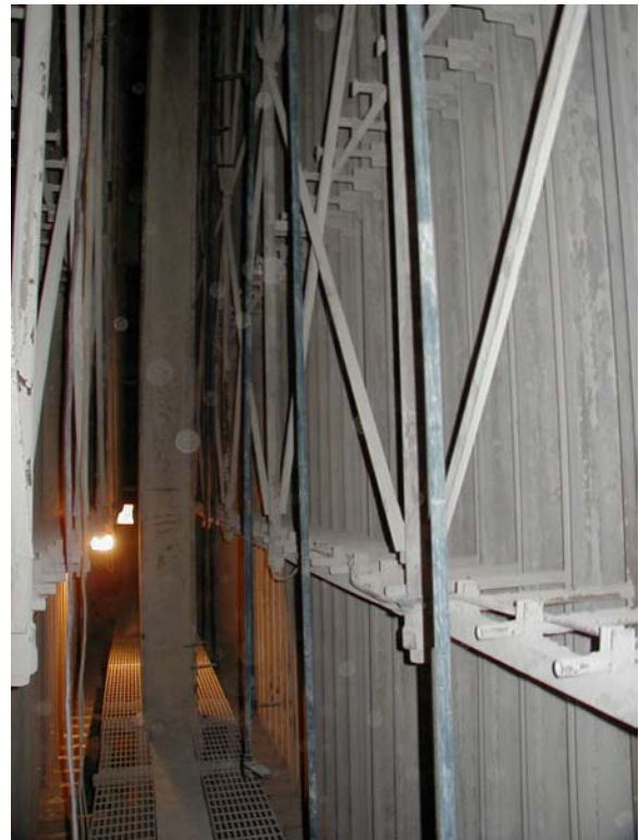
Figure 5. Injection Grid Between ESP Fields.
